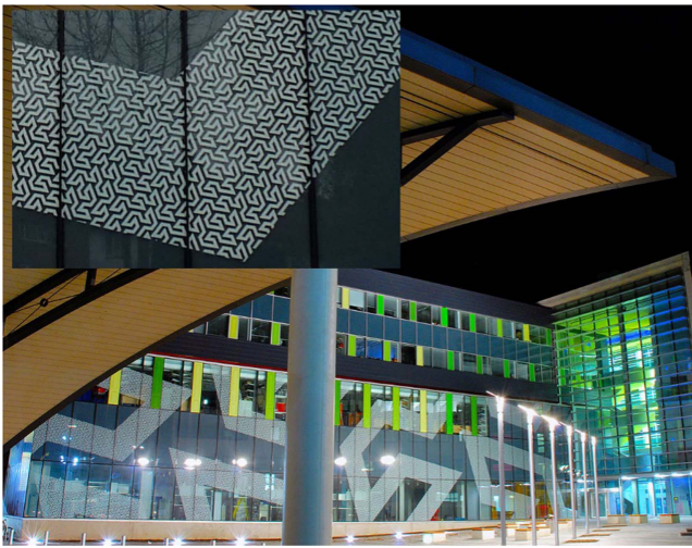
Figure 2. University of Southampton Mountbatten Building, which hosts the Optoelectronics Research Centre and the Centre for Photonic Metamaterials, and stands on the site of the Southampton Silicon Foundry; it is arguably the only building in the world covered with a metamaterial design. The inset (top left) shows a fragment of the planar-chiral fractal metamaterial pattern developed within the first metamaterial research grant ‘Optical manifestations of planar chirality’ awarded to NIZ in 2002. The pattern was developed by A Potts, D Bagnall and N I Zheludev, and was fabricated on a silicon wafer at the Southampton Silicon Foundry shortly before fire destroyed it. Its design was the inspiration for the pattern on the building.
